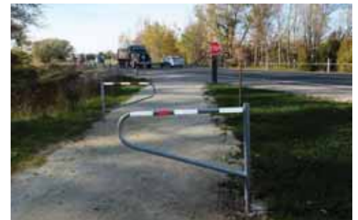
Bollard gating has been installed on both sides of the Georgian Trail where it crosses Highway 26 east of Thornbury.
