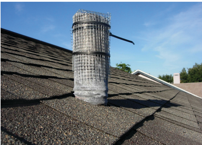
Figure 7. Cover roof vent pipes with hardware cloth to prevent entry into buildings by Cuban treefrogs Credits: Steve Johnson, UF/IFAS
