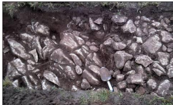
Edge of the road marked by the trowel The sheet bedrock is on the left and is a whiter, grittier stone than the roadstone, which is rough limestone with soil on the right of this picture
