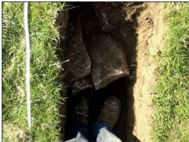
Large edging stones "pitching" supporting the terracing
