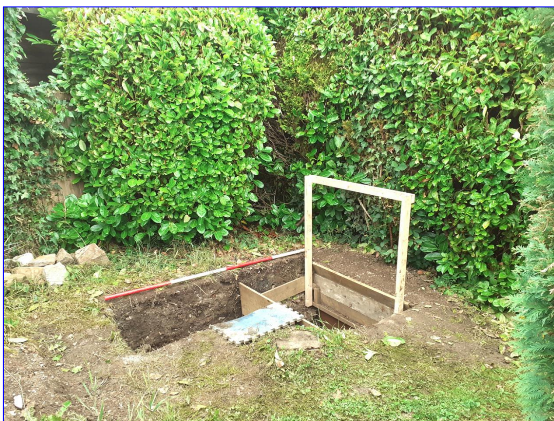
Trial trench 2 with additional shuttering being constructed
