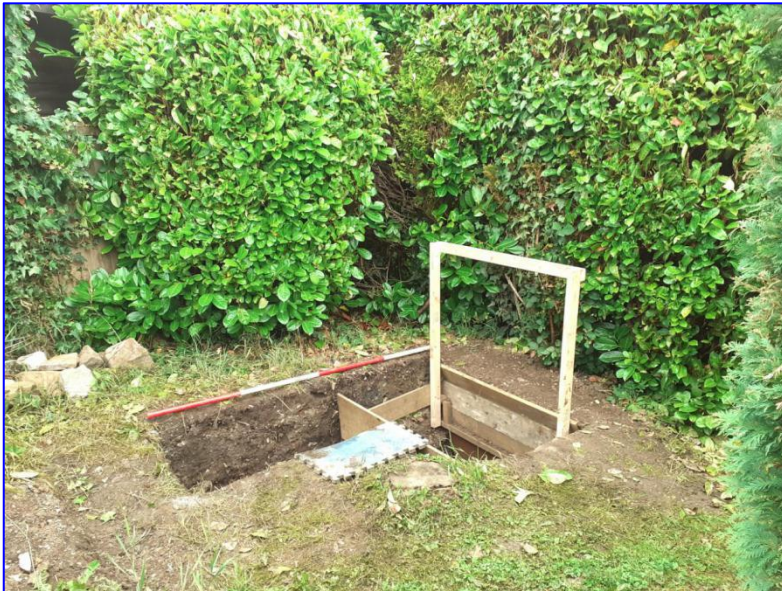
Trial Trench 2 general view looking north-west
