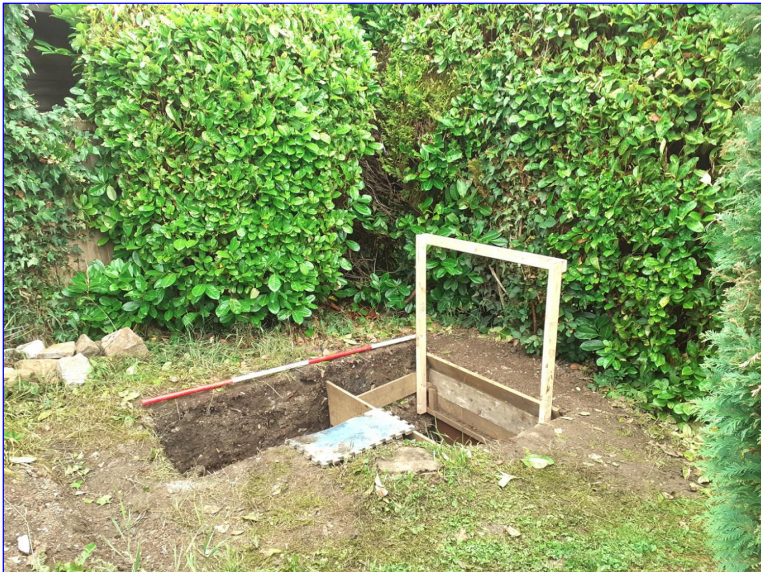
Trial trench 2 with additional shuttering being constructed
