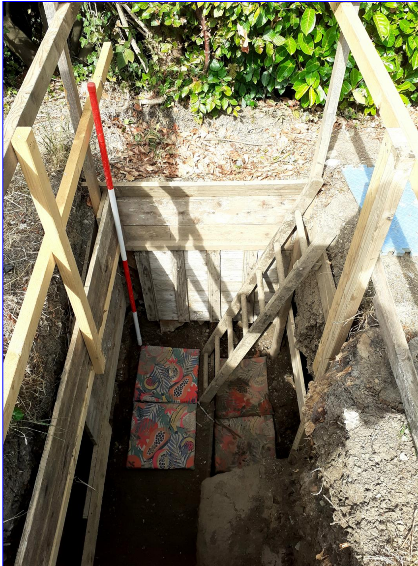
Trial Trench 2 looking north, showing shuttering and fall arrest (cushions)
