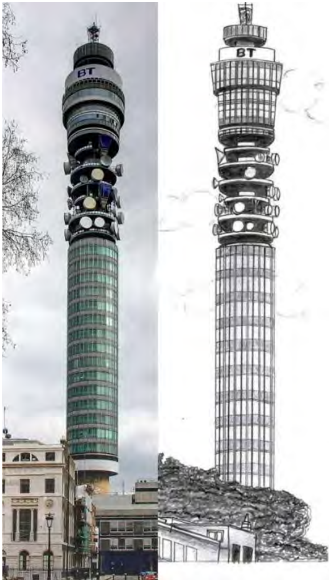
Eric Bedford + CR Yeats: GPO Tower (later BT Tower ) 1965. By the mid-Sixties, real architecture was catching-up with Archigram's visions. Designed to carry microwave transmitters to link London into the GPO (General Post Office) UK-wide Microwave network, with a revolving restaurant near the top - it was inspiring, and somehow very cool - we were on top of the telecoms revolution...
