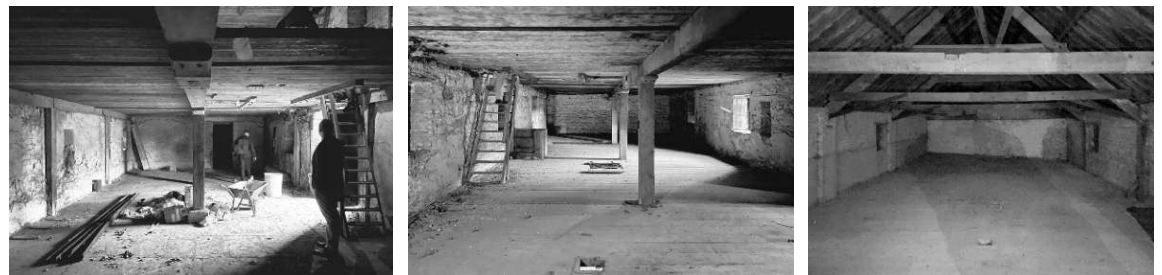
Ground, first and second floors (from left to right) at present in Young's Stores. Note the flagstone floors, timber central beam and columns and thick structural floorboards.
