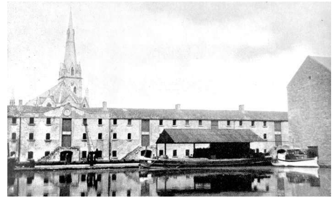
The store building along the West edge of the site with the pediment with a plaque at its centre. This was clearly axially organised with the Harbour inlet as a composed design. Angela Rolt 1946
