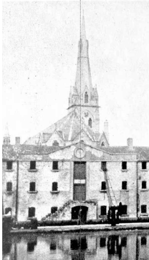
The break-front centre bay of the linear store building on the west of the Harbour complex (a redline highlighting the centre axis of the pediment and round plaque).
