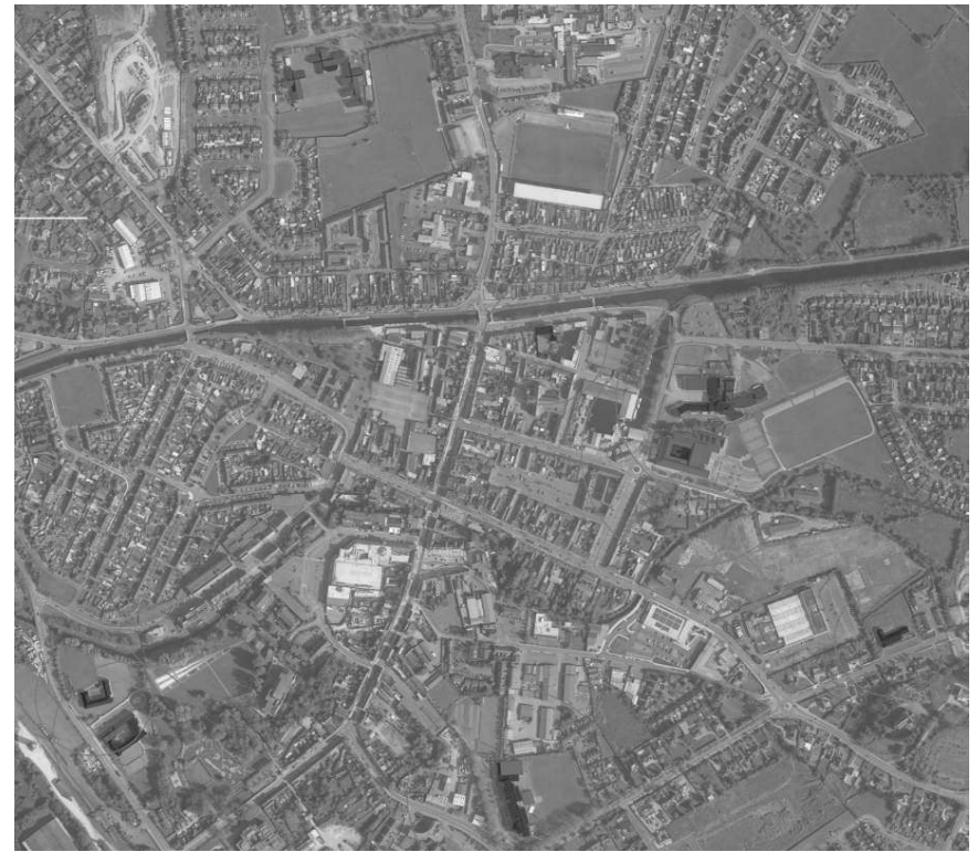
The schools of Tullamore indicated on an aerial photo of the town - a number of which are directly adjacent to the Harbour & Canal Spur.
