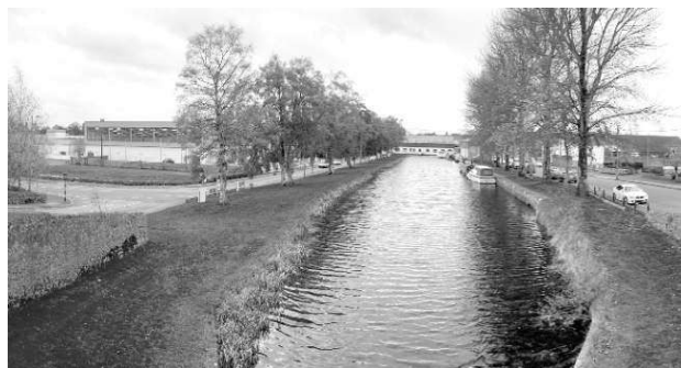
The Canal Spur from the Whitehall (Bury) Bridge
