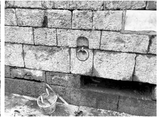
Photos of careful repair and replacement of eroded limestone blocks within a canal lock chamber at Mespil Rd, Dublin.
