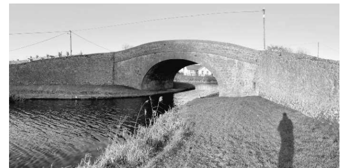
The Whitehall (Bury) Bridge viewed from the East embankment.
