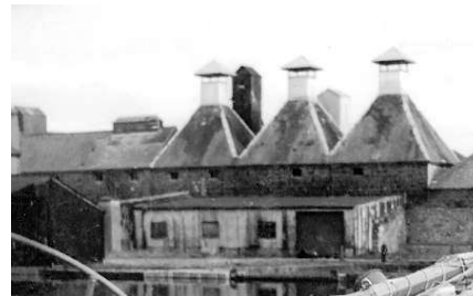
Photograph from within the harbour of the cowls in Egan's Maltsters (now demolished) on Harbour St. Photograph by Kevin Donaghy.
