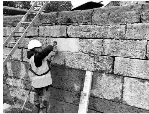
Photos of careful repair and replacement of eroded limestone blocks within a canal lock chamber at Mespil Rd, Dublin.
