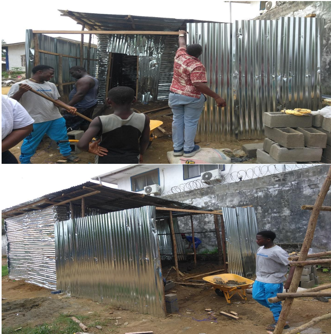
Construction of the AB Tolbert Road plastic Buying Station CNCL Photo credit April 30, 2026 Catherine D.
