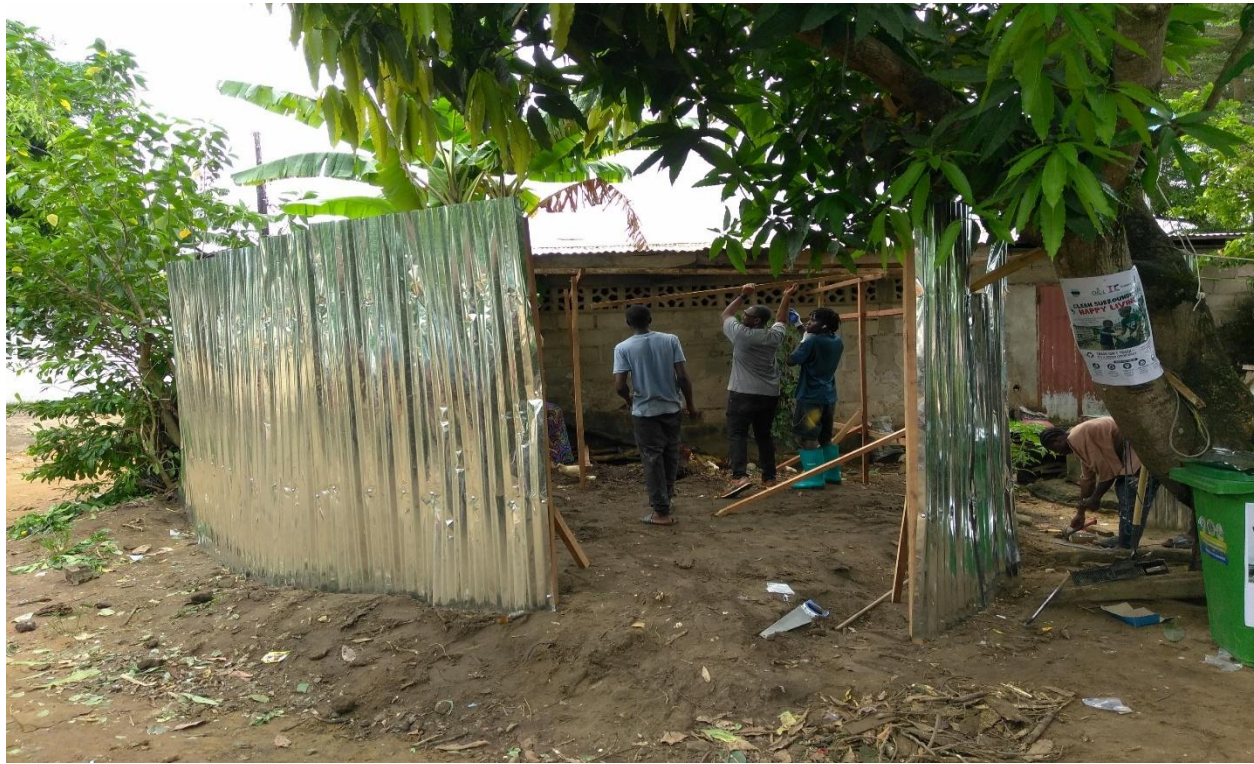
Construction of the Duport Road plastic Buying Station CNCL Photo credit May 12, 2026 Catherine D.
