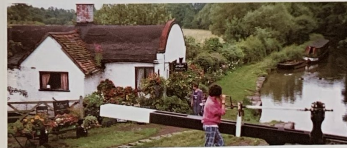
A typical barrel-roofed cottage on the Stratford-on-Avon canal.
