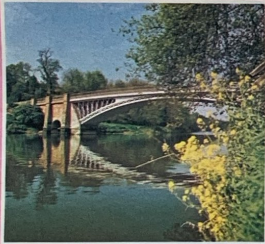
Telford's bridge over the Severn at Holt
