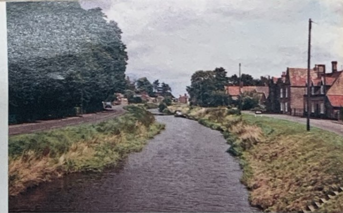
Upwell, Well Creek (Fen Waterway)
