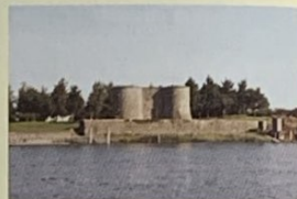
Tower at Banagher
