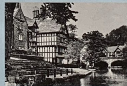
A fine view of the Canal Architecture at Worsley.
