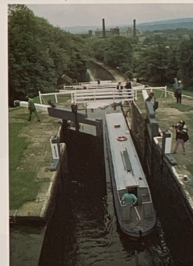
3 Bingley Five Rise. A "staircase" of locks lifts the canal 60 ft up the side of the Aire Valley on the Leeds & Liverpool Canal. Opened to the ringing of church bells two centuries ago, it leads to 16 lock-free miles of cruising - and Ilkley Moor!
