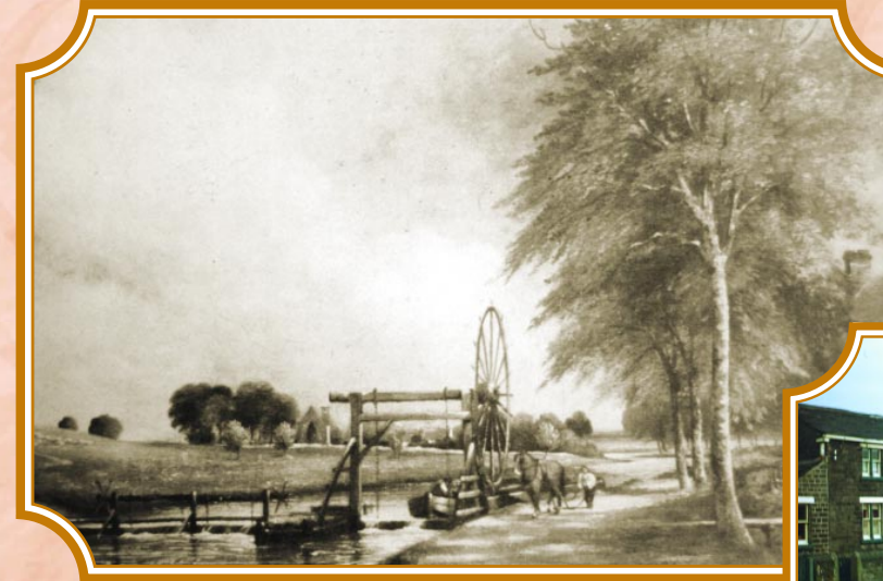
On the earliest river navigations, 'flash' locks were used. These were removable gaps in a weir through which the boats passed. They were not popular with the mill owners as they wasted water. Vertically lifting gates were introduced later by engineers from the Low Countries to reduce water loss.
