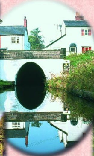
▲ Preston Brook Tunnel
