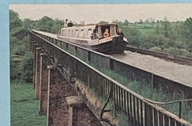
Edstone Aqueduct, Stratford-on-Avon Canal
