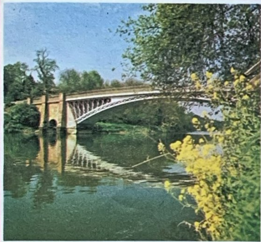
Telford's bridge over the Severn at Holt
