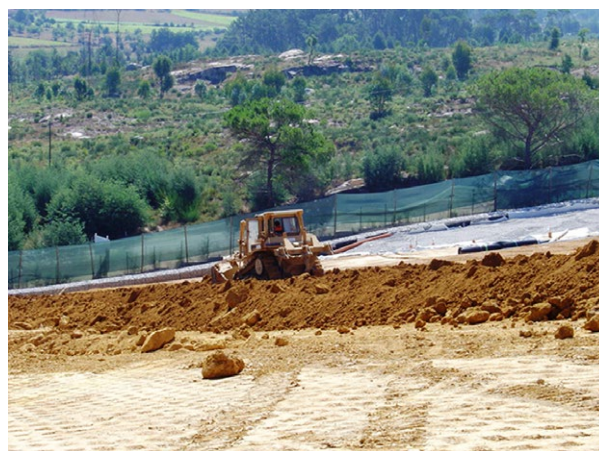
Figure 14. Remediation of legacy uranium tailings (Urgeirica Mine, Portugal) placing a cap of geotextile membrane and several soil layers to confine radioactive uranium mill tailings.
