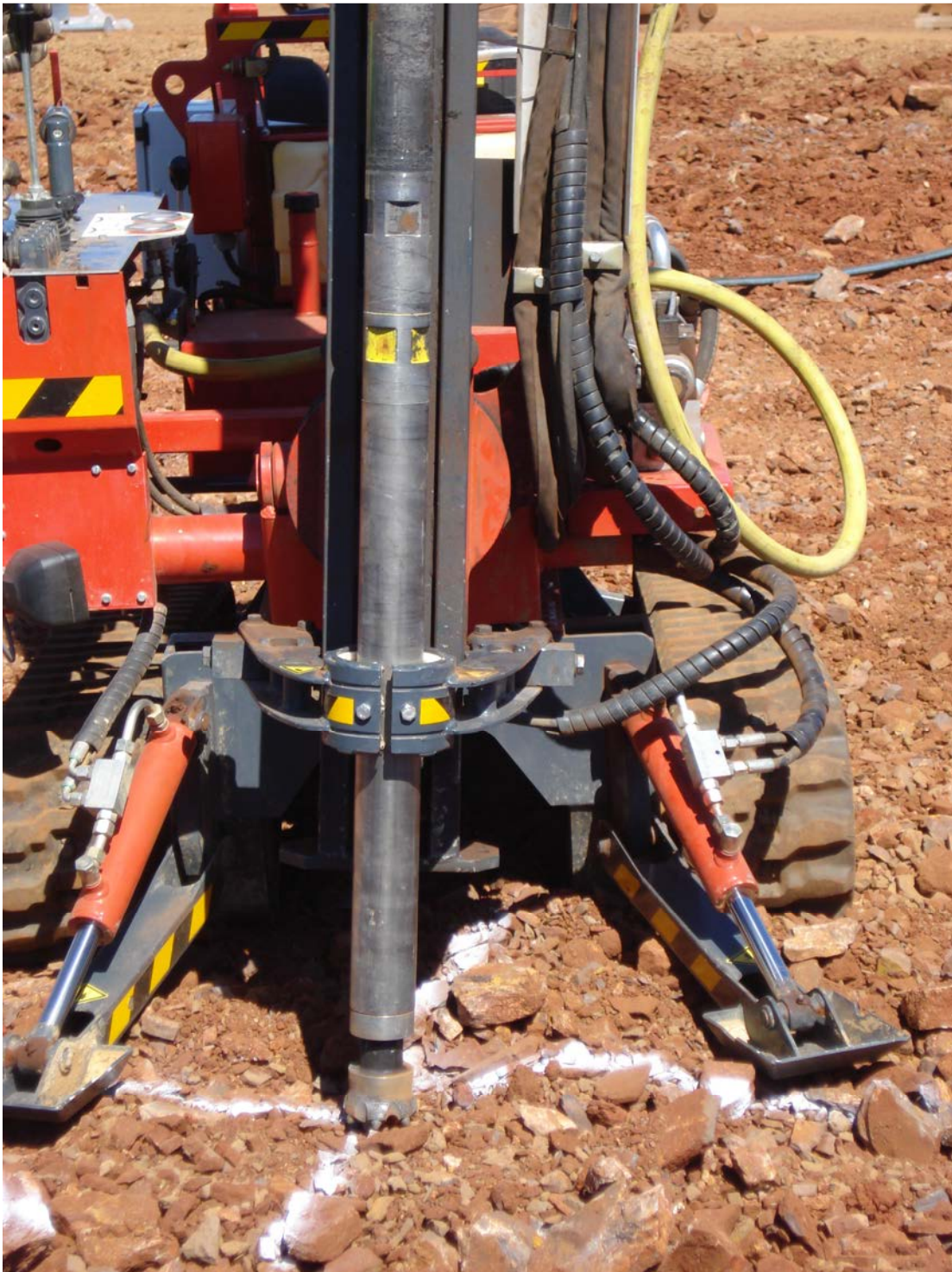
Photo 1. Pre-drilling in rock
