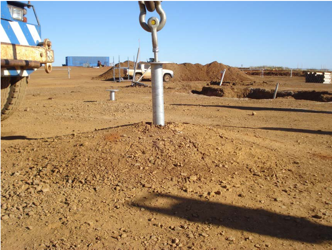
Photo 5. Pullout Test 6 in compacted fill, photo taken immediately before failure
