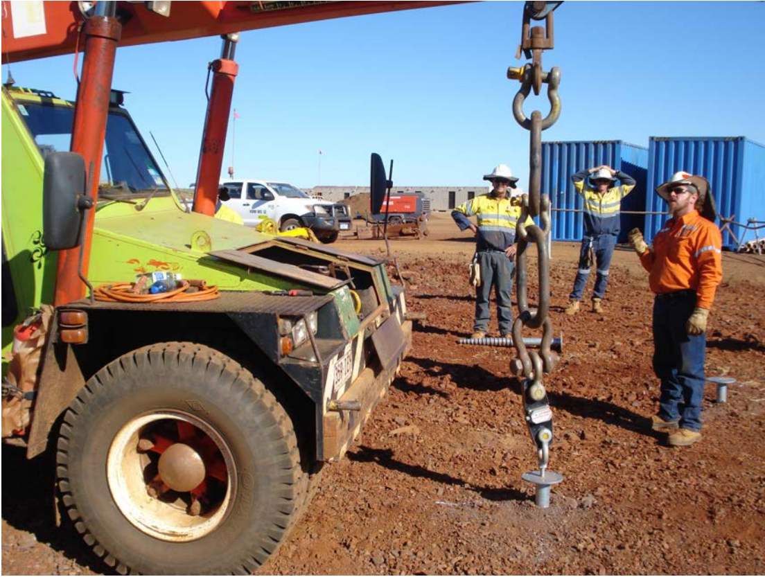
Photo 3. Pullout Test 2 in rock
