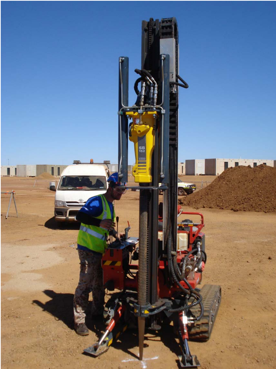
Photo 2. Pre-drilling in compacted fill
