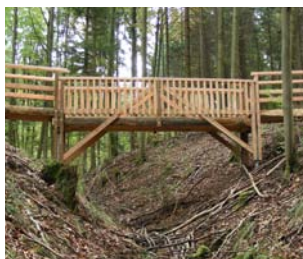
Pedestrian bridge / Boardwalk
