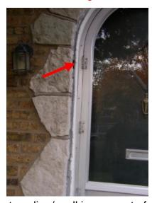
Suggest sealing/caulking as part of routine maintenance at all penetrations through the walls.
