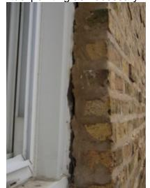
Caulking of siding and windows at cracks, crevices, any openings, penetrations is needed on all windows and doors
