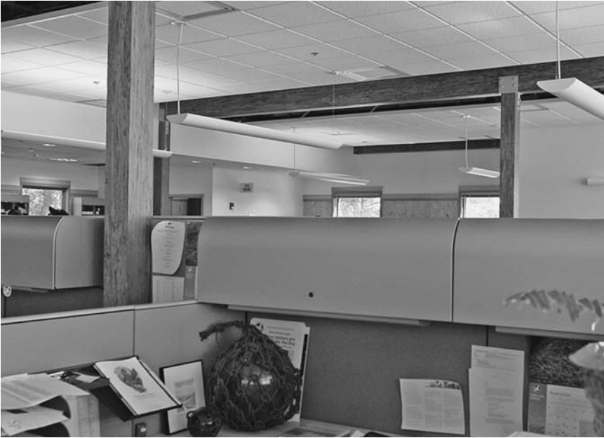
FIGURE 19.5 Indirect lighting provides high quality diffuse illumination in the Chesapeake Bay Foundation's Merrill Building. Photo by Carl Bovill.
