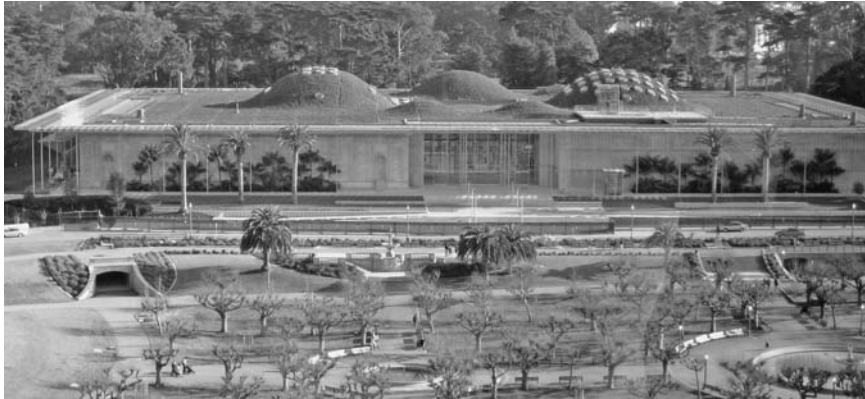
FIGURE 25.2 The green roof on the California Academy of Sciences Building in Golden Gate Park, San Francisco, California. The architect was Renzo Piano, and the green roof was designed and installed by Ran Creek in 2008. Photo by Carl Bovill.
