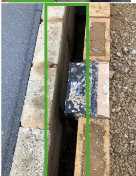
Photographs should show the generic insulation type\* (e.g. mineral wool, PIR) installed below the DPC and should match what has been used in the psi value models.
