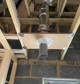
Photographs should show that mechanical ventilation ductwork in unheated spaces e.g. cold roof spaces is insulated.
