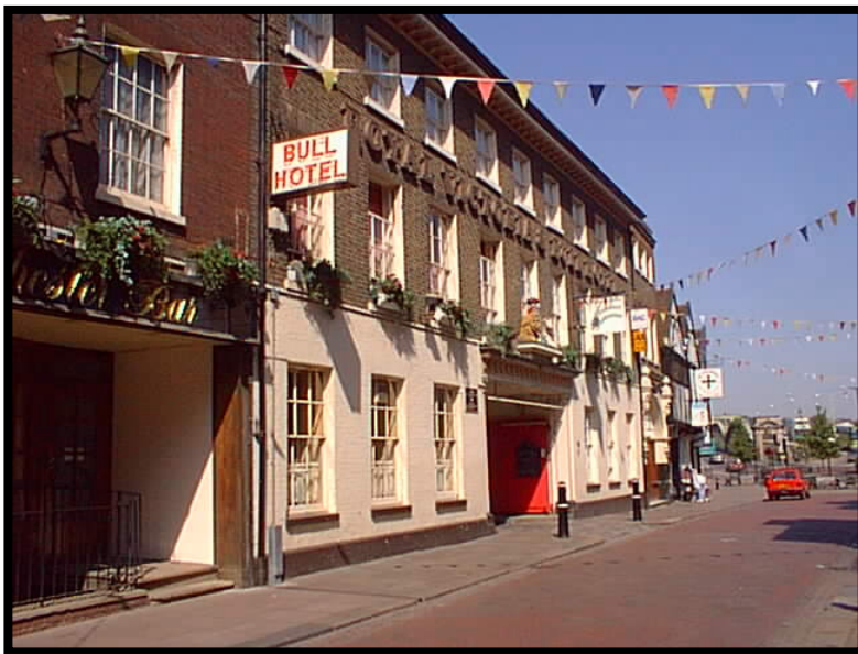
A coaching inn of Samuel Wickenden's times still stands in Rochester High Street. The entrance was wide and high enough for six-horse teams to enter the inn. Beyond the red car may be seen the arches of the steel bridge.
