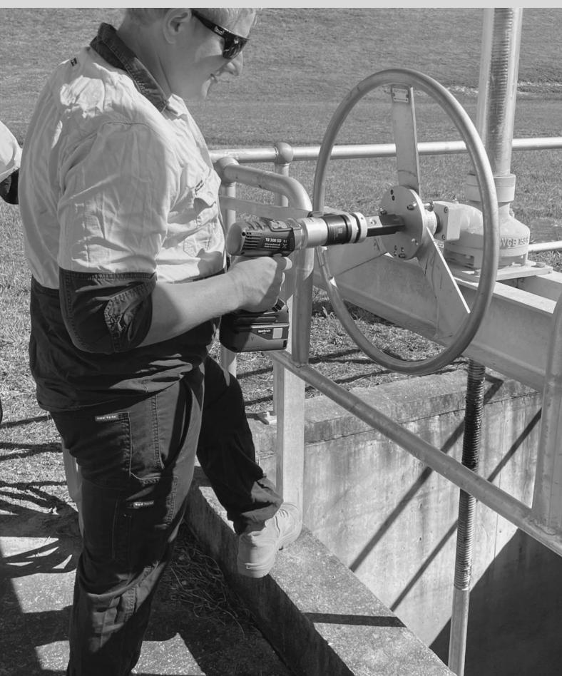
**Cordless Portable Valve Actuator System**
