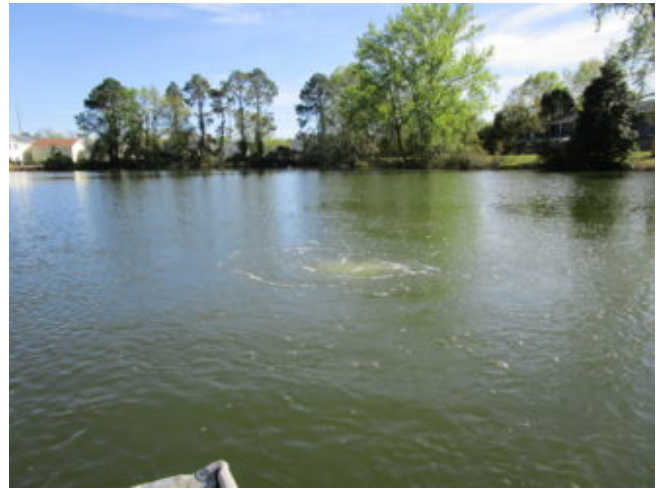
A bottom diffuser is used in this stormwater pond to help circulate the water column, preventing stratification and dissolved oxygen concerns in the pond. Photo courtesy The Lake Doctors, Inc. C. Guinn Wallover, ©2020, Clemson Extension
