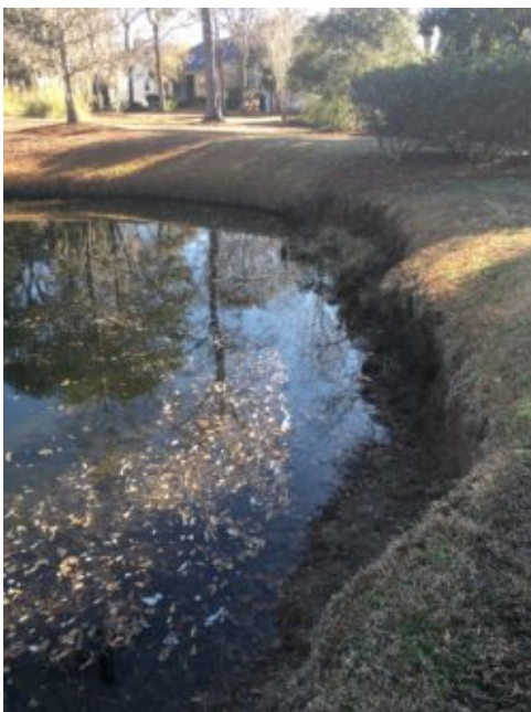
Erosion and the undercut of pond banks are common pond maintenance concerns. These issues can often be attributed to the presence of turfgrass along the shoreline, which lacks the tolerance to moist soil conditions and erosive wave energy
