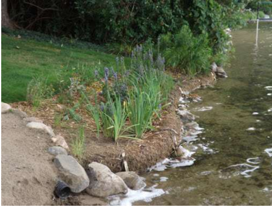
Example of a Shoreline Repaired With Coir logs and Wetland Plants
