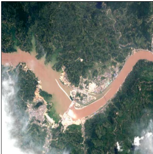
Three Gorges Dam, China, 2003
