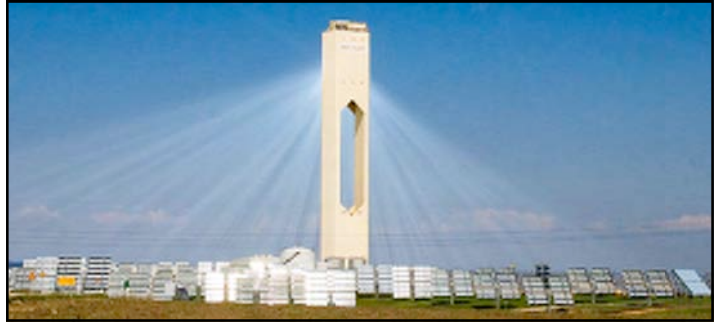
Fig. 25 Southern view of Spain's Power Tower, PS10, in Seville; source: beyondzeroemissions.org
