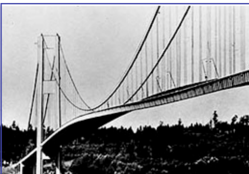
Figure 20. The Tacoma's Narrows Bridge, which collapsed in 1940 due to the phenomenon of aeroelastic flutter. Source: Humdingerwind.com
