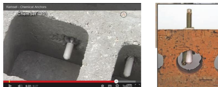
Figure 20 © Ramset ChemSet 101 and nylon sleeve
