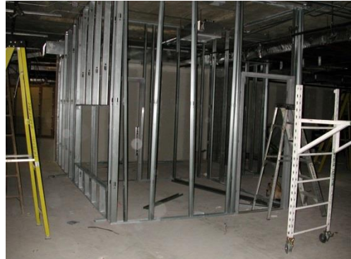
Figure 42 © Wikipedia Steel Frame Wall
