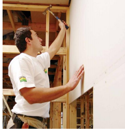
Figure 2 © Boral Timber frame hollow wall with plasterboard
