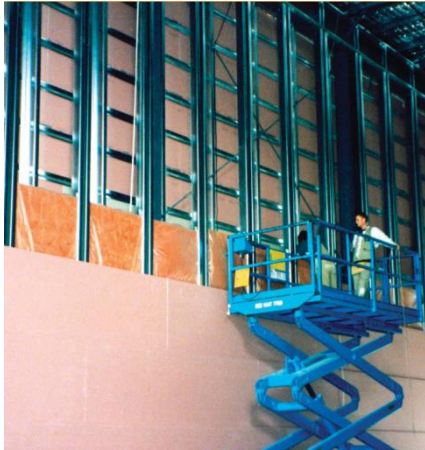
Figure 1 © Boral Steel frame hollow wall with plasterboard
