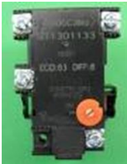
Bimetallic Disc Type Thermostat ©NMTAFE 2014
