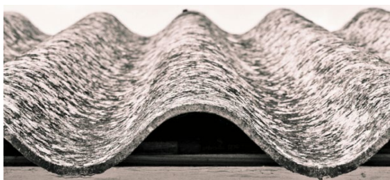
Asbestos cement corrugated sheeting
