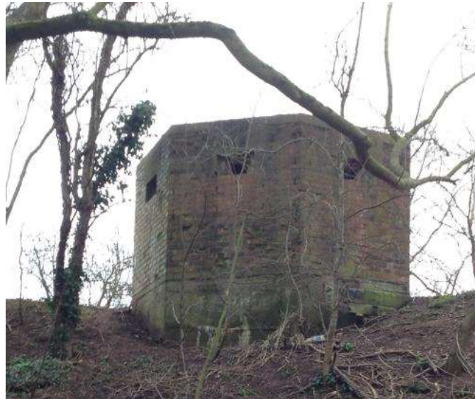
Figure 11 Pillbox, near Radford Semele Bridge
