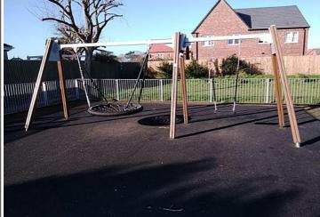
**Finding:** The seat clearance from finished surface level to the underside of the seat is too low when measured in its most onerous position and does not meet the requirements of BS EN 1176 Part 2
