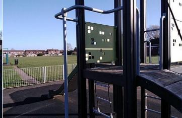
**Finding:** The firemans pole is less than 350mm from the platform and does not meet with the recommendations of BS EN 1176 Part 1
