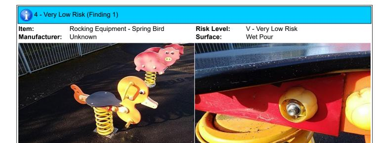
**Finding:** There is/are bolt cap covers missing or damaged on the item
