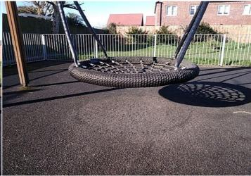
**Action:** Install seats to a minimum height of 400mm for Group Swing Seats
