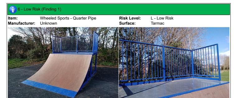
**Finding:** The height of the barrier is less than 1200mm and **Action:** Monitor - No remedial work recommended fails the requirements of BS EN 14974
