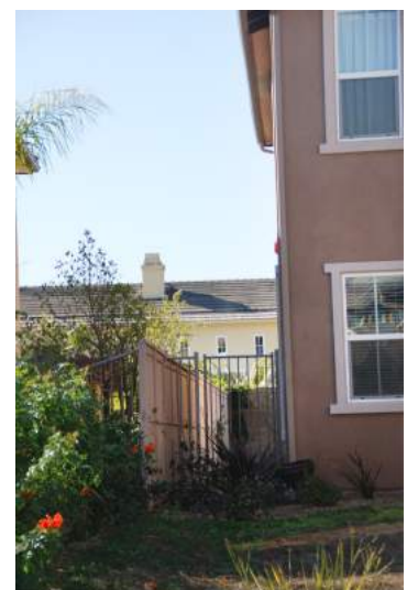
A gate made from noncombustible materials should be used where a connection is made to the house. Source: firecenter.berkeley.edu/bwmg/attachments-1.html
