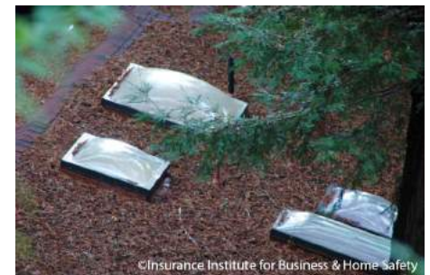
Flat (top photo) and domed (bottom photo) skylights. Note propensity for debris to accumulate on top of flat versus domed skylights.
