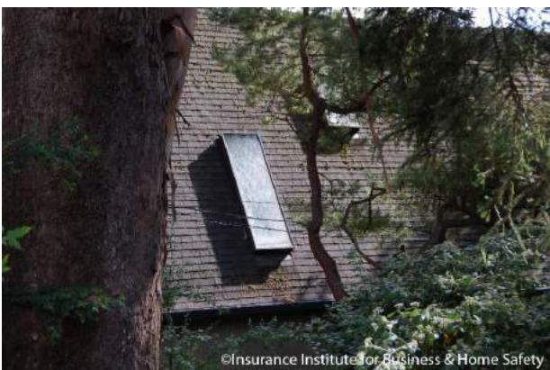
Skylight on a steep-slope roof. Radiant heat exposure from burning vegetation or building would be more of a problem with steeper sloped roofs.
