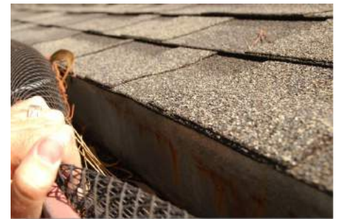
Gutter with integrated drip edge. Source: firecenter.berkeley.edu/bwmg/gutters.html
