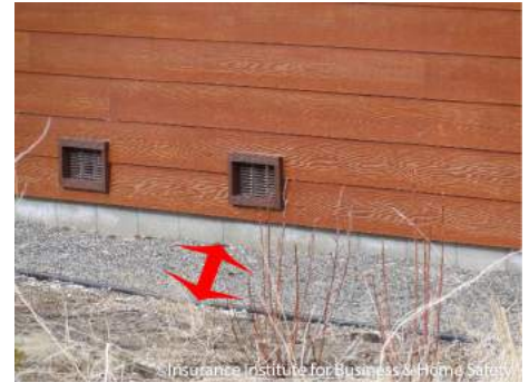
A noncombustible zone around a home in the Lake Tahoe Basin. In this case, requirements related to water runoff and protection from wildfire align.
