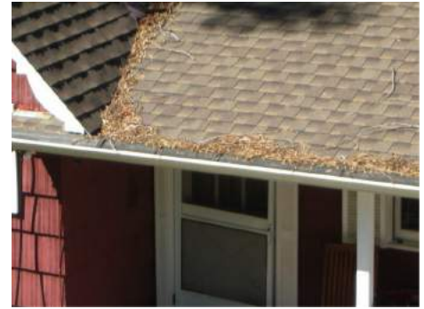
Debris accumulation on roof covering behind gutter cover device. Source: firecenter.berkeley.edu/bwmg/gutters.html
