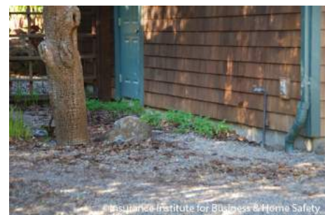
Clearance between the ground and the start of the siding should consistently be at least 6 inches.
