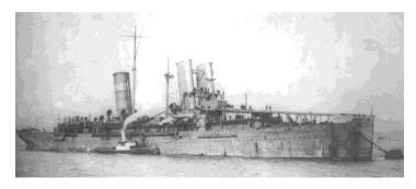
November 1915 and April 1916. The flight deck was extended to a length of 245 feet and Campania now carried seven Short 184 torpedo bombers and three or four smaller fighters or scouts. A Type 184 made its first takeoff from the flight deck on 3 June 1916, also using a wheeled trolley. This success prompted the Admiralty to order the world's first aircraft designed for carrier operations, the Fairey Campania and the
