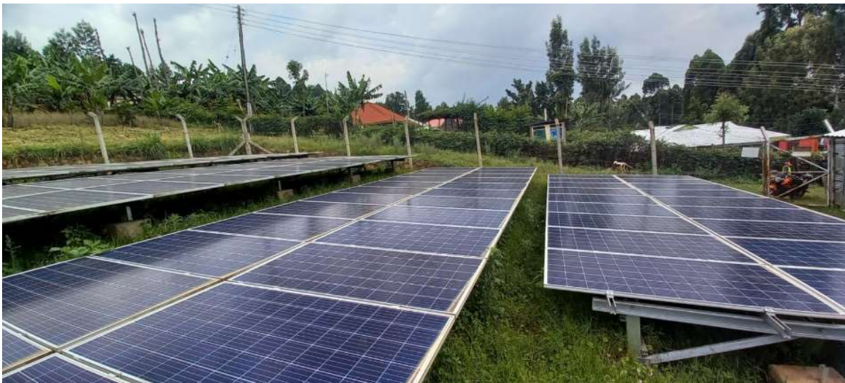
Photo 9: Solar mini grid at Gionseri B, Kisii County Photo credits: Rosebella Nyumba
