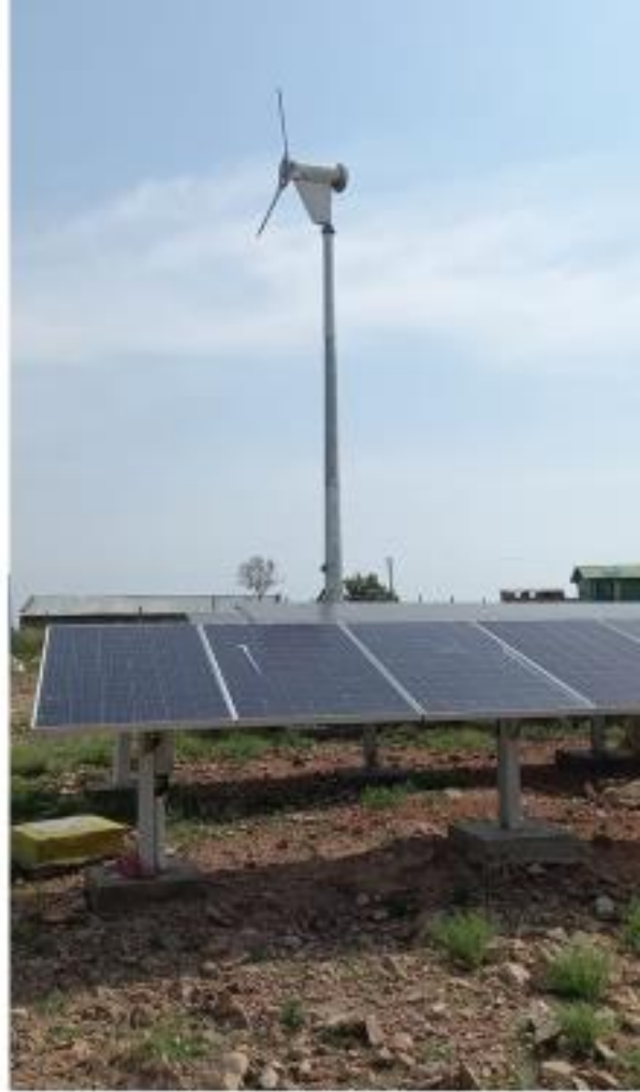
Hybrid Mini grid(Solar and Wind) In Ndenda Island,.
