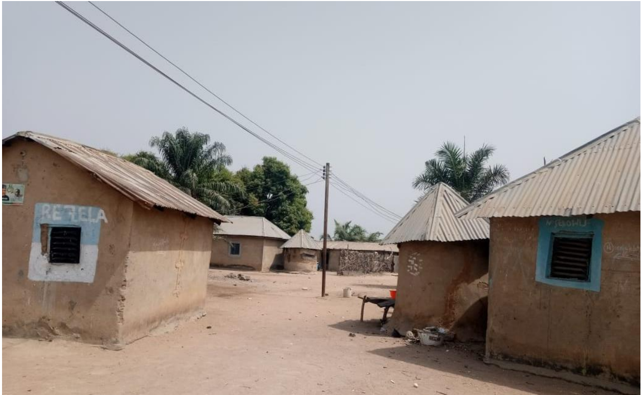
Figure 2. Rije Community biogas mini grid and community
