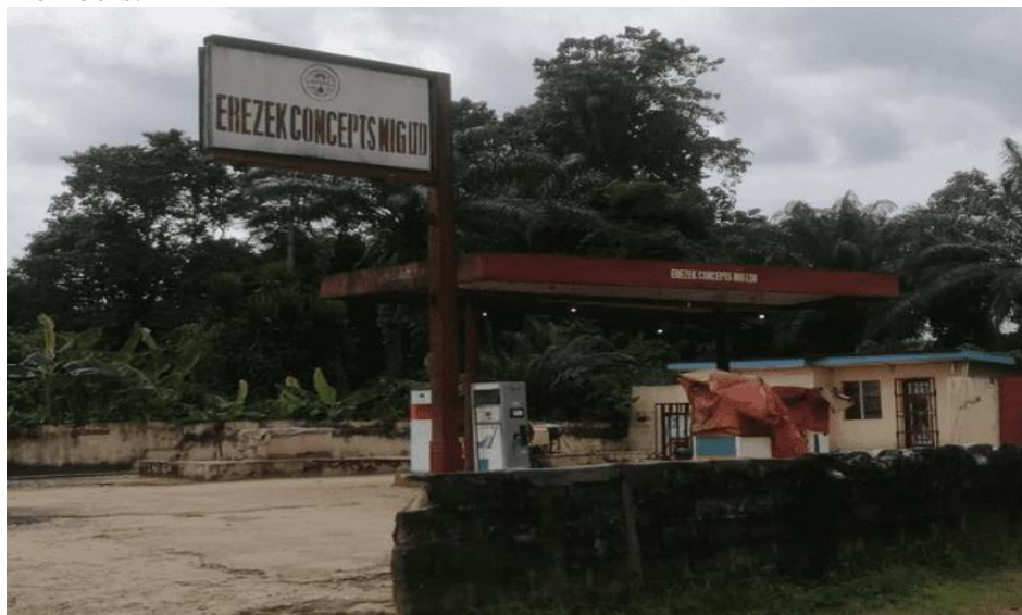
Figure 8: Filling station powered by energy from the mini grid in Ozuzu community
