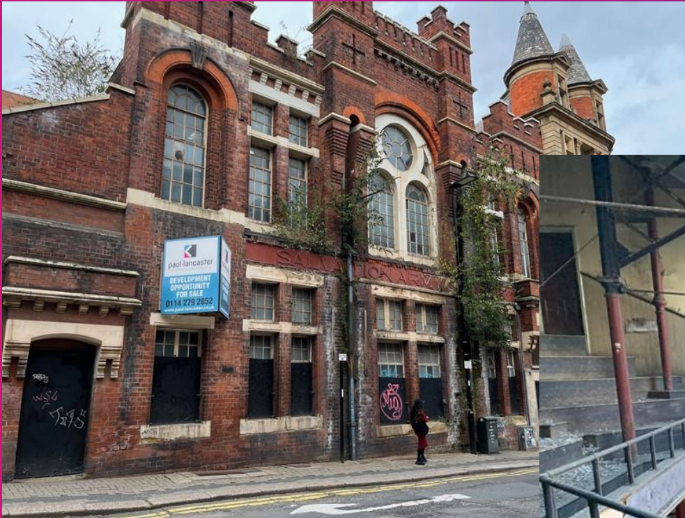
Cross Burgess Street
