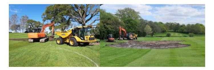
Once cleared, the excavation of the pond could begin utilizing the versatility of Hitachi zx180 excavator with it Engcon roto-tilt attachment and the Hydrema 912FS 180-degree swivel 10 ton articulated dump truck with floatation tyres.
