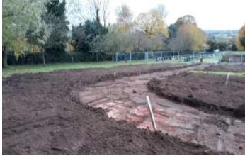
Once cleared, the excavation of the road could begin utilizing the versatility of our Takeuchi TB290 excavator and Thwaites 4.5-ton hydrostatic site dump truck with floatation tyres.
