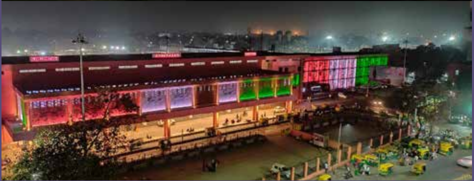
Ahmedabad Railway Station Lighting Project Completed By Surya
