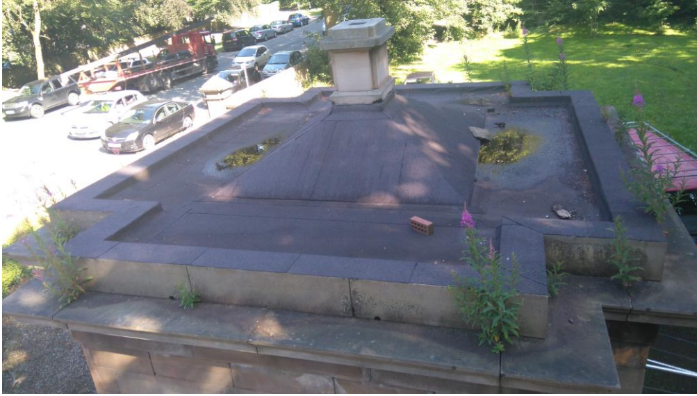
Photograph 5: Roof Covering Lodge 1
