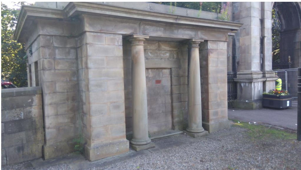
Photograph 4: Front Elevation of Lodge 1
