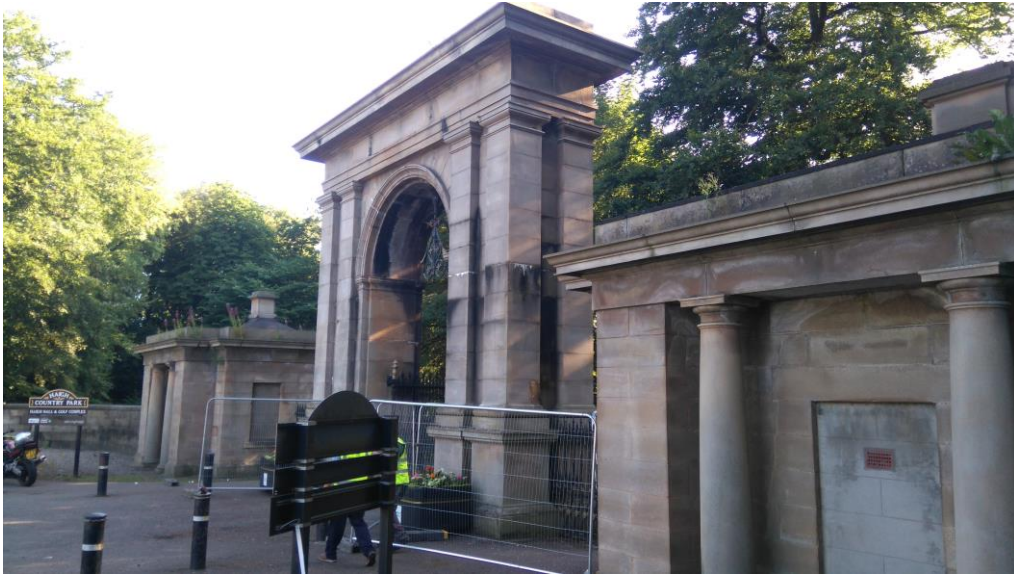
Photograph 1: Front Elevation Of Archway and Lodges
