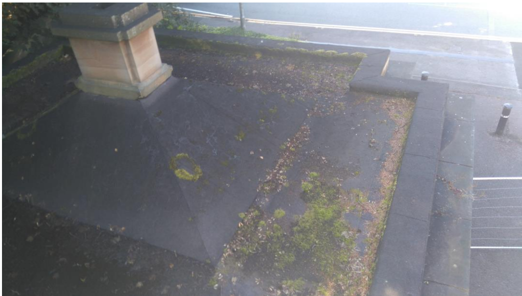
Photograph 6: Roof Covering Lodge 2
