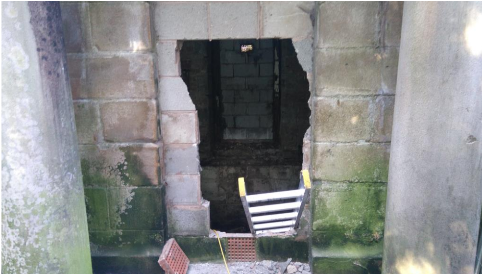
Photograph 11: Lodge 1 - Opening Up Of Doorway
