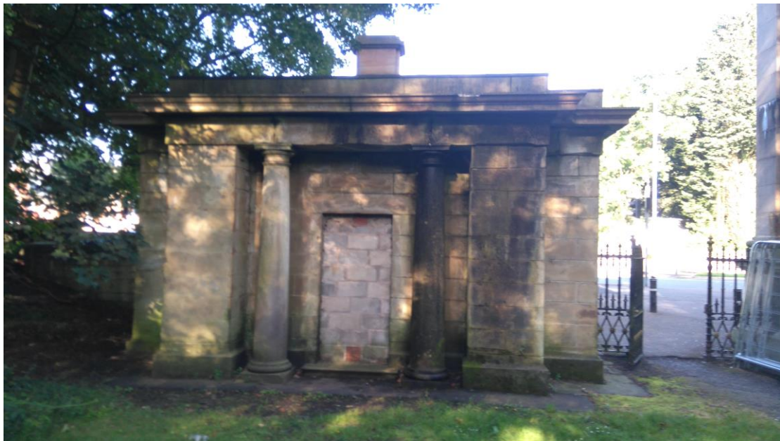
Photograph 2: Rear Elevation of Lodge 2
