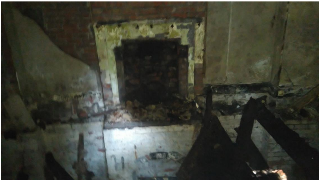
Photograph 16: Lodge 2 - Fire Place
