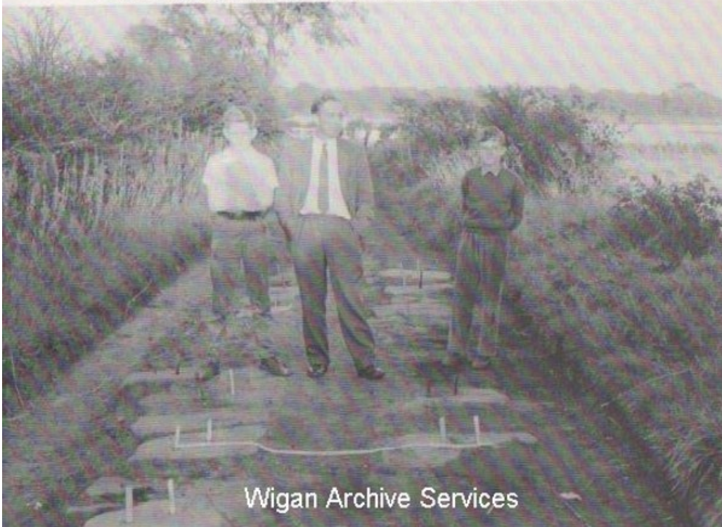
29 Clarke's wagon road at Winstanley, showing the stone sleeper-blocks. On here ran Dalglish's Yorkshire Horse , Lancashire's first steam locomotive
