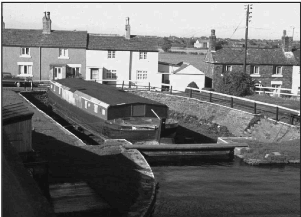
The drydock at Top Locks in the late-1970s, with the Juno under repair. Formerly one of the coal boats belonging to John Parkes & Sons, at this time it usually provided accommodation alongside the sports field at Parbold.
