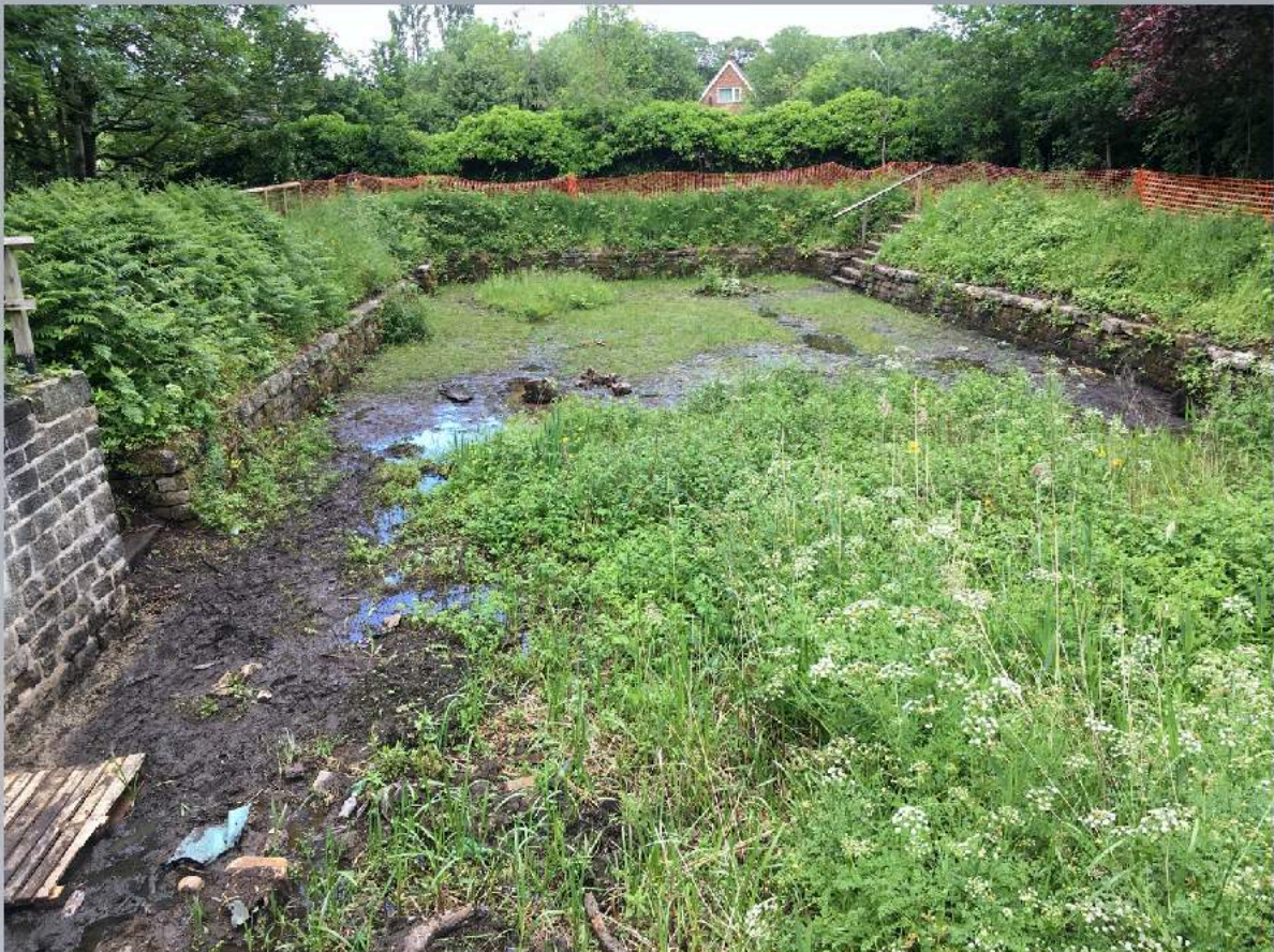
Basin June 2019 - Grass starting to grow in cleared area
