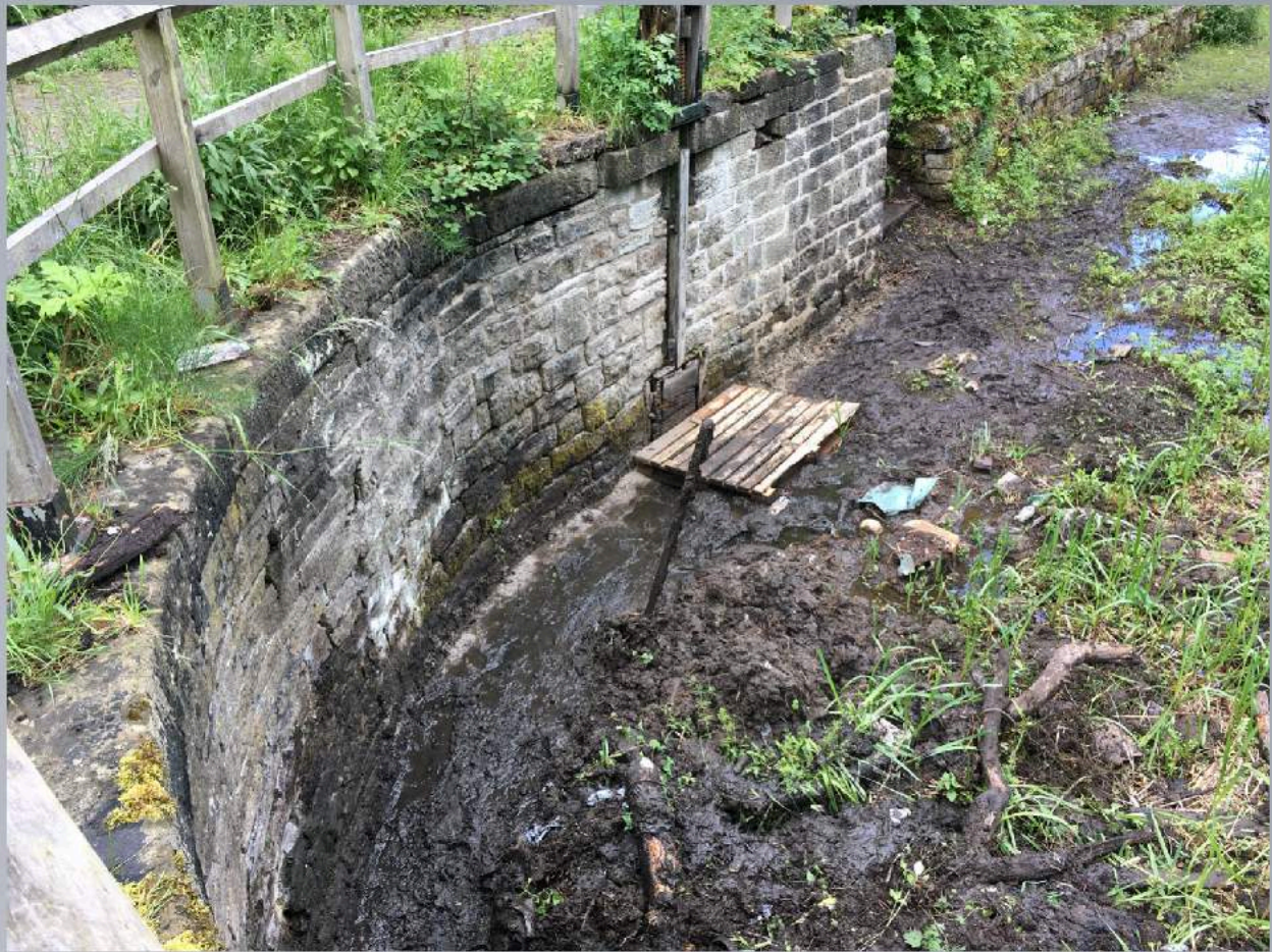
Lime Mortar pointing of the Dock Wall June 2019
