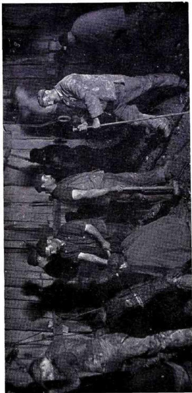
Plate I. SINKING BY HAND DRILLING, WIGAN, 1900
